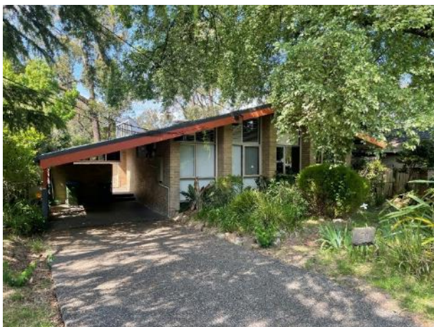
Figure 2 20 Rawson Court, Ringwood East
