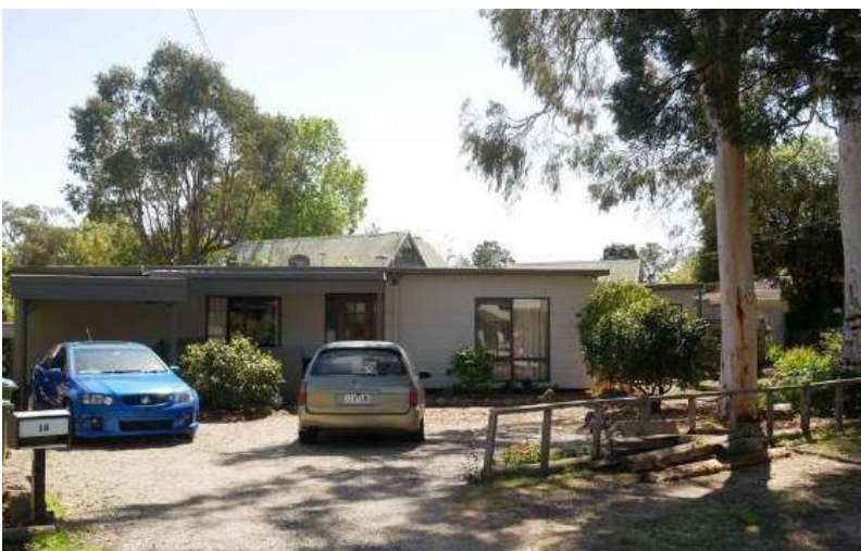
Figure 8 18 Valerie Court, Heathmont
