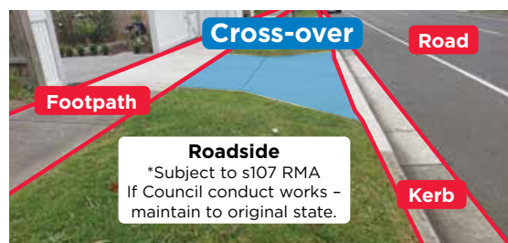
Figure 3 Example of Vehicle Crossing Demarcation
