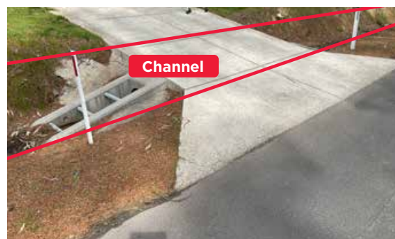
Figure 6 Example of channel transverse Vehicle Crossing
