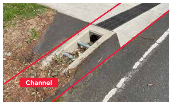
Figure 5 Example of channel transverse Vehicle Crossing
