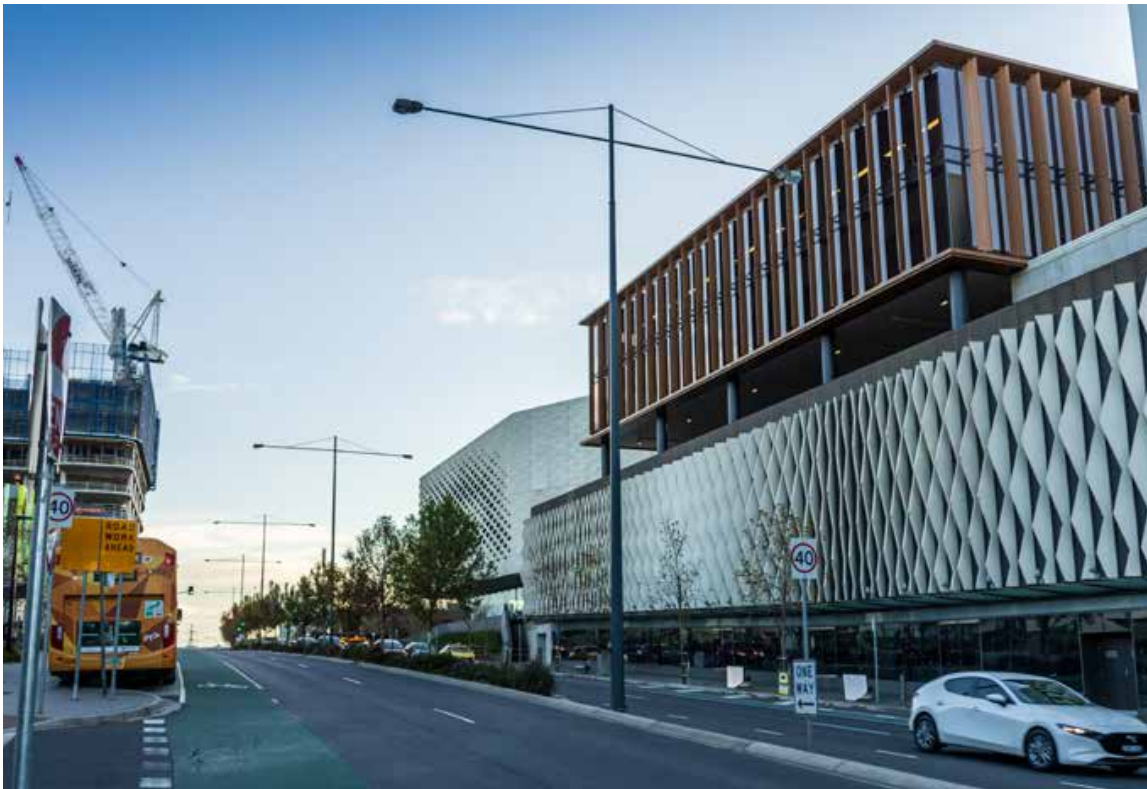
Maroondah City Council's civic and administrative offices are located in Realm at Ringwood Town Square
