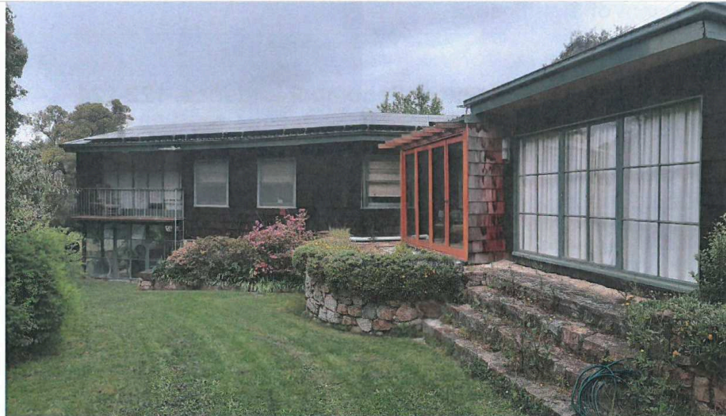
Composite panoramic photograph of the Heathmont Road frontage, taken by City of Maroondah, October 2020. Note stone terrace, steel-framed window wall to living room (right), projecting sunroom with timber-framed glazed doors, and master bedroom wing (far left) with another steel-framed window wall, balcony and glazed infill below.
