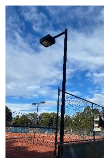
Low mast halogen Croydon TC
