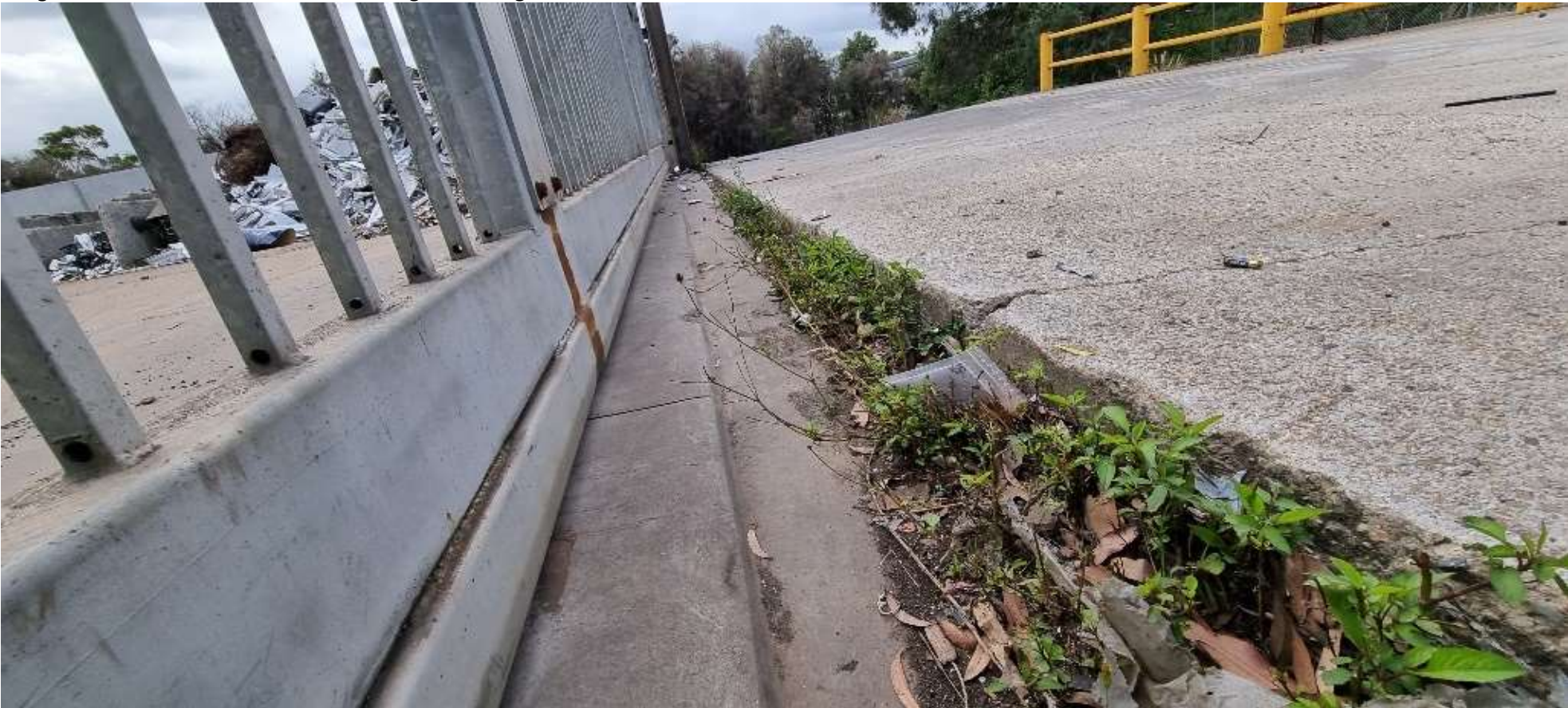
Image 5. Raised channel at the base of the gate in Image 4
