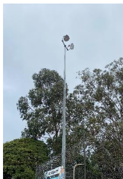
High mast halogen East Ringwood TC
