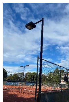
Low mast halogen Croydon TC
